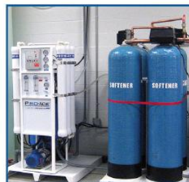
Pro Ice Reverse Osmosis Water Treatment
