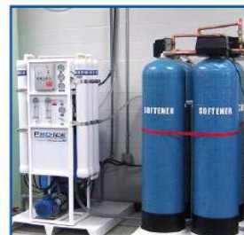
Pro Ice Reverse Osmosis Water Treatment
