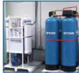
Pro Ice Reverse Osmosis Water Treatment
